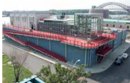
Figure 1 – SHARON® demonstration plant at Wards Island Wastewater Treatment Plant in Manhattan, New York (Image courtesy of M2T Technologies)
