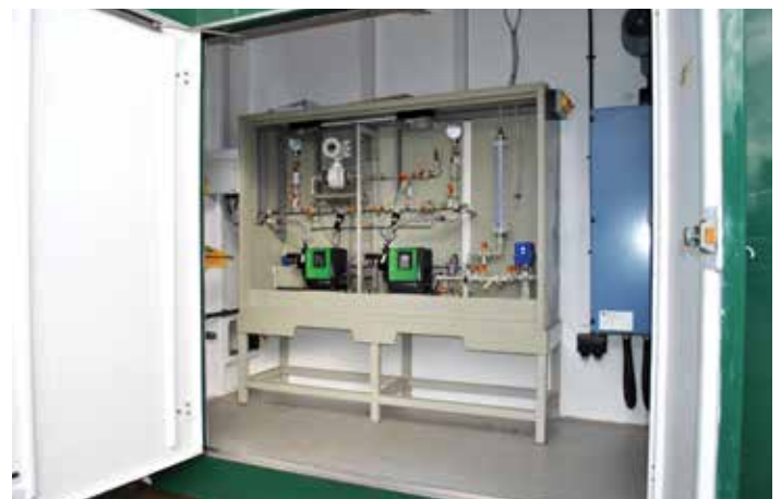
A dosing skid being installed onsite prior to being enclosed by a kiosk with a control system
