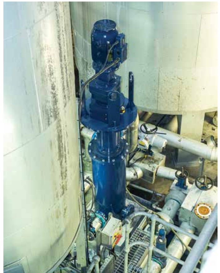
seepex vertically mounted pump
