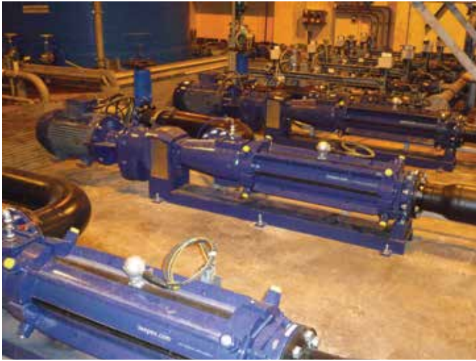
seepex SCT pumps feed centrifuge
