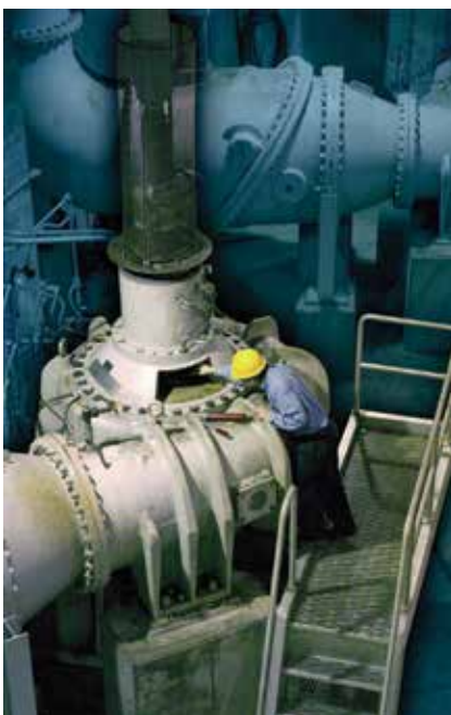
Figure 2: Large pumps – Ideally Sealed with Split Seals
